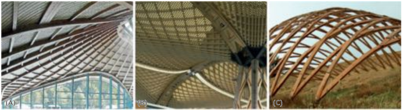
Fig. 1. Timber Gridshells using geodesic planks. (A) The ribbed Gridshell in Bad Dürkheim was built with a primary grid along the principal curvature lines and a diagonal cover of geodesic planks. (B) The Expo Hannover Gridshell (by Natterer & Herzog) combines laminated geodesic ribs with a diagonal geodesic substructure. (C) The deployable geodesic Almond Gridshell (by Soriano) was designed to allow a flat assembly and kinetic erection process.
