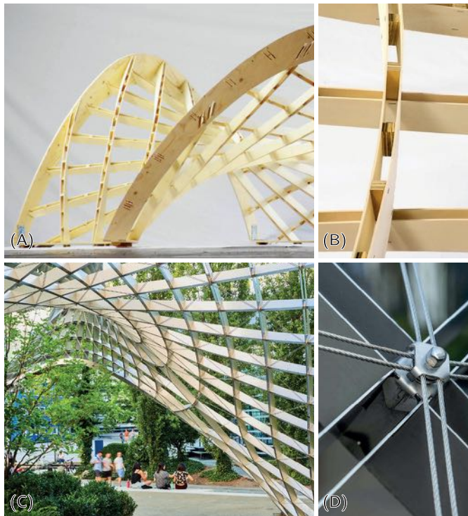
Fig. 2. Gridshells using asymptotic networks. (A,B) The first asymptotic timber prototype was developed at the TUM in 2016, using double lamellas of laminated poplar and square timber studs. (C,D) In 2017, the Inside/Out Pavilion was built out of stainless steel lamellas, with repetitive 90-degree joints, and was braced with diagonal pre-stressed cables.
